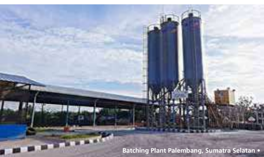
Batching Plant Palembang, Sumatra Selatan •
